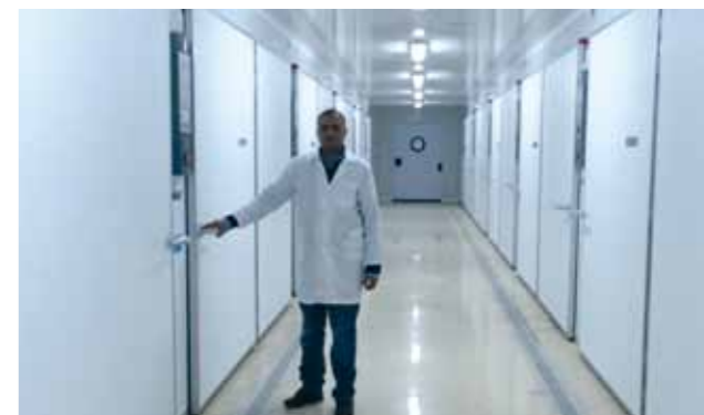
Setter corridor of the new hatchery.
